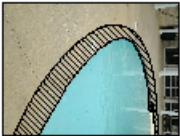
EAST END OF POOL AREA OF CONCRETE REPAIR
