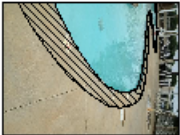
NORTH END OF POOL AREA OF CONCRETE REPAIR
