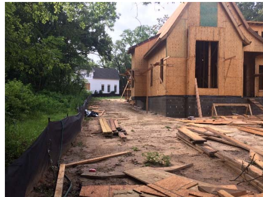
Northern property line looking east
